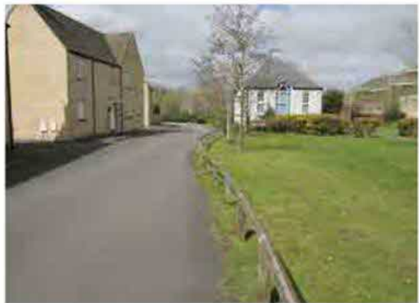
Figure 8.5 Shallow swale on a site with shallow groundwater, Witney, Oxfordshire (courtesy EPG Limited)
